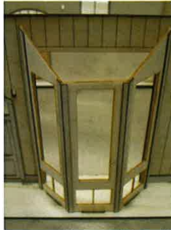
Applied Corner Supports (F) and (K)
